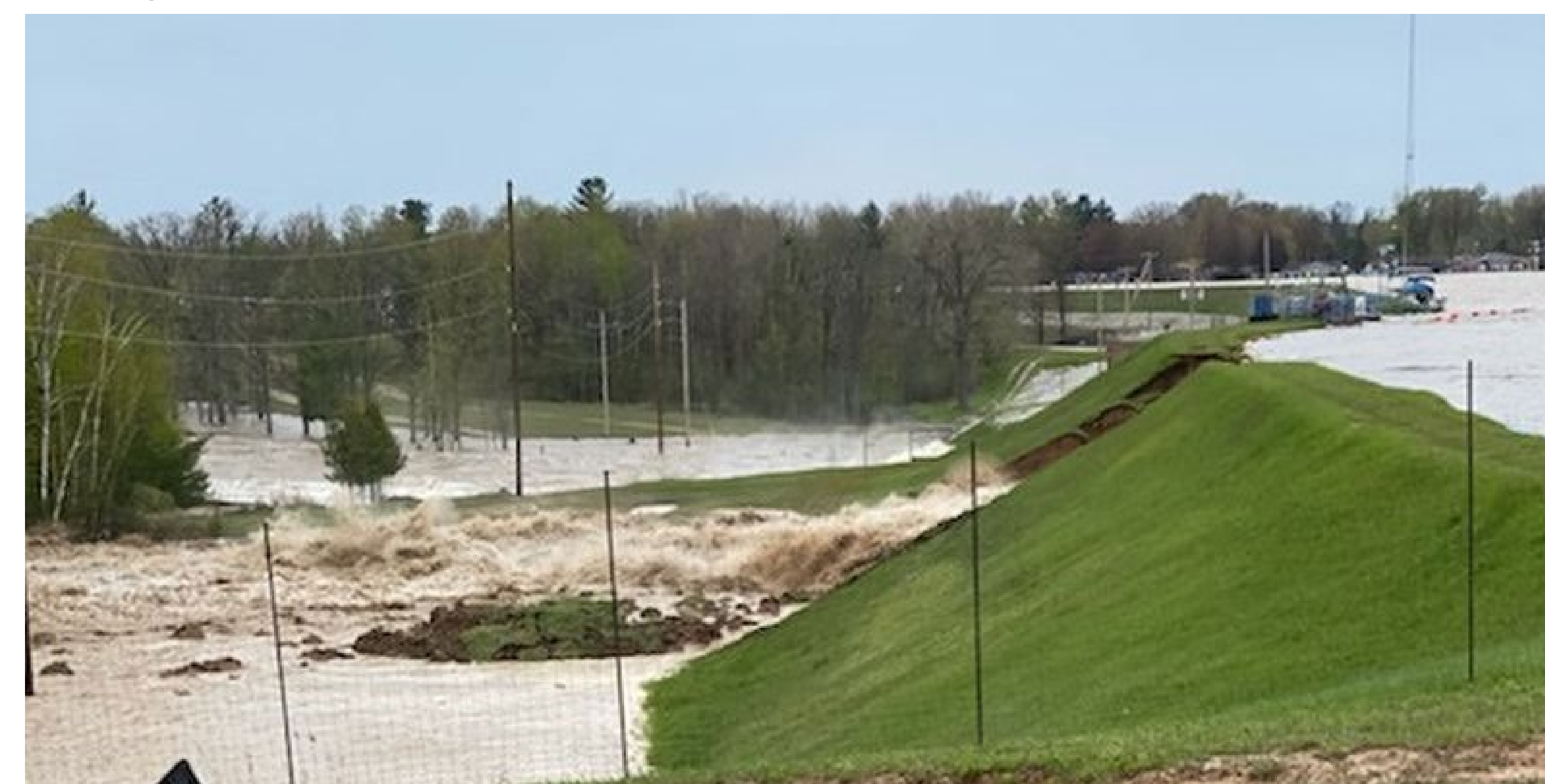
When the Edenville Dam failed during this rain event, it emptied 21.5 billion gallons of water downstream and emptied the lake in one hour.
