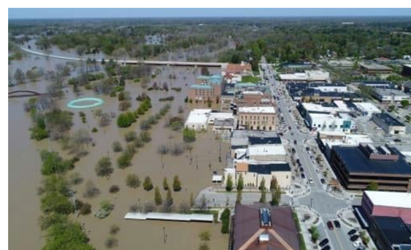
Severe flooding following the failure of the Edenville and Sanford Dams.
