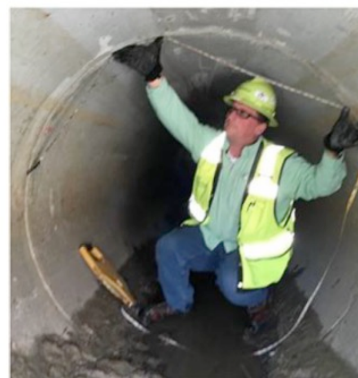
FIG. 1 Person Entry Inspection
