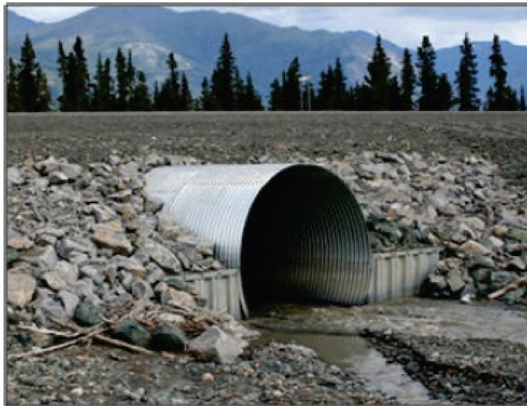
Figure 5.19. Unanchored thin edge projecting.
