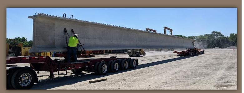
COMPARED TO CAST-IN-PLACE STRUCTURES, PRESTRESS CONCRETE BEAMS CAN BE INSTALLED FASTER WITH FEWER REQUIREMENTS.
