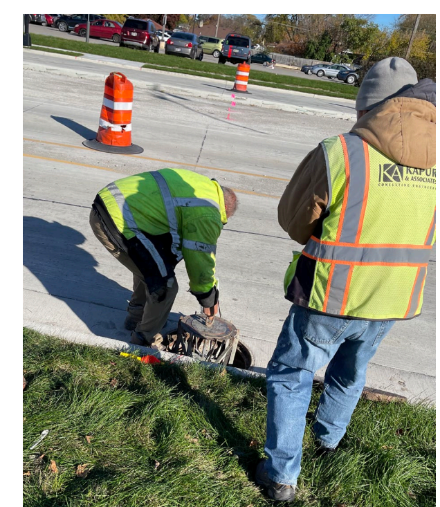
Mandrel lowered to test 24” HDPE pipe
