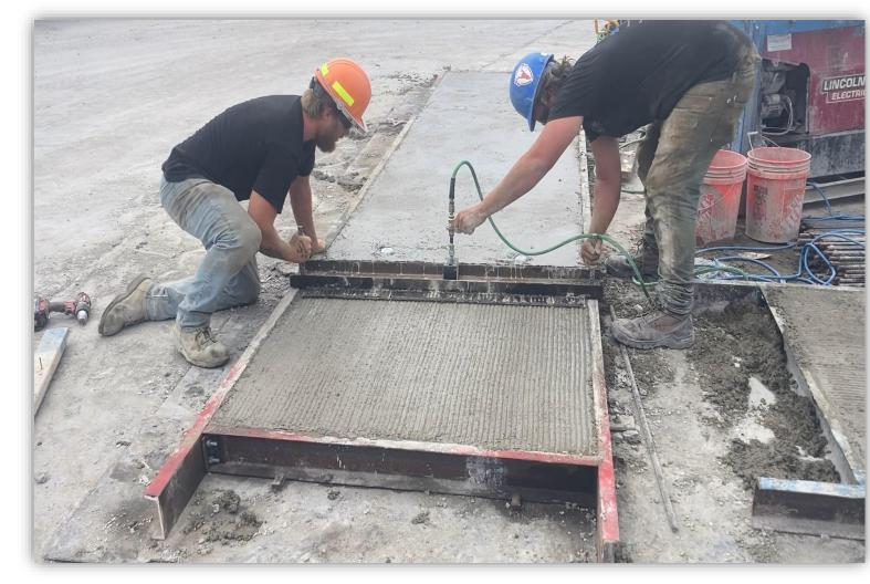
Roll the screeding tool down the length of the form for a consistent and high-quality anti-slip finish every time!
