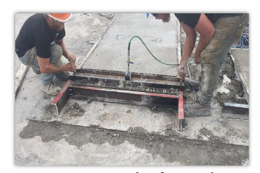
Once set on the form, the screeding tool has centering lugs to ensure it is centered and straight, as well as rollers to ensure it maintains straightness while working down the length of the form
