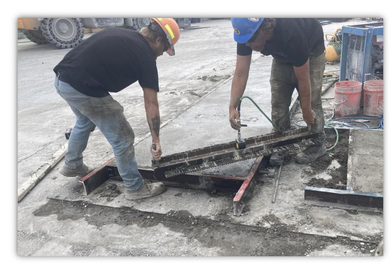
Simply connect air hose to the vibrator and place on the form. In this example it's a boat launch ramp, which needs aggressive grooves for tire traction in wet and icy conditions.
