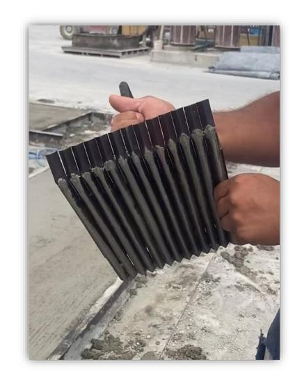
Air powered vibrator mounted on custom grooved screeding tool vibrates the screed while floating it along surfaces, bringing paste to the surface and forming neat, clean, straight, and uniform grooves. With the help of the custom touch-up tool, we can be even more certain every piece will look it's best!
