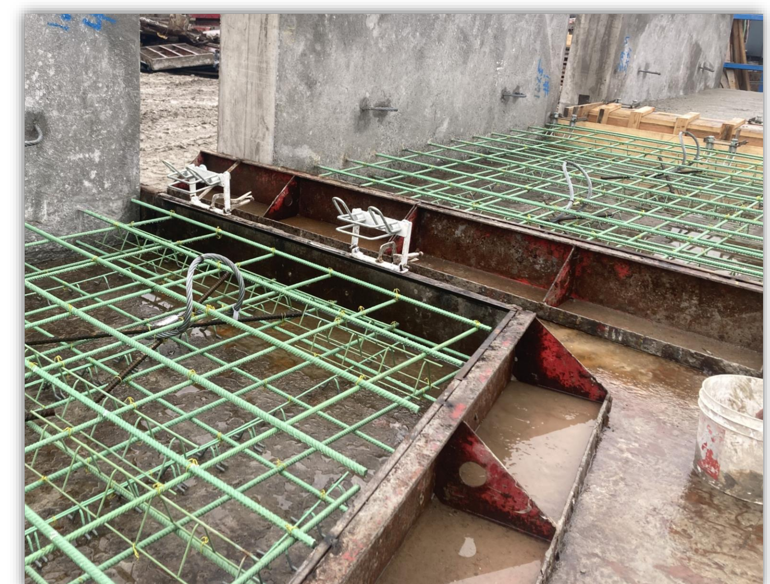
Once position is verified during pre-pour inspection, the anchor is able to be hinged out of the concrete and out of the way for concrete placement. This is done without having to relocate the anchor bracket, or unbolting the anchor, ensuring the anchor is returned to the exact position that was verified.
