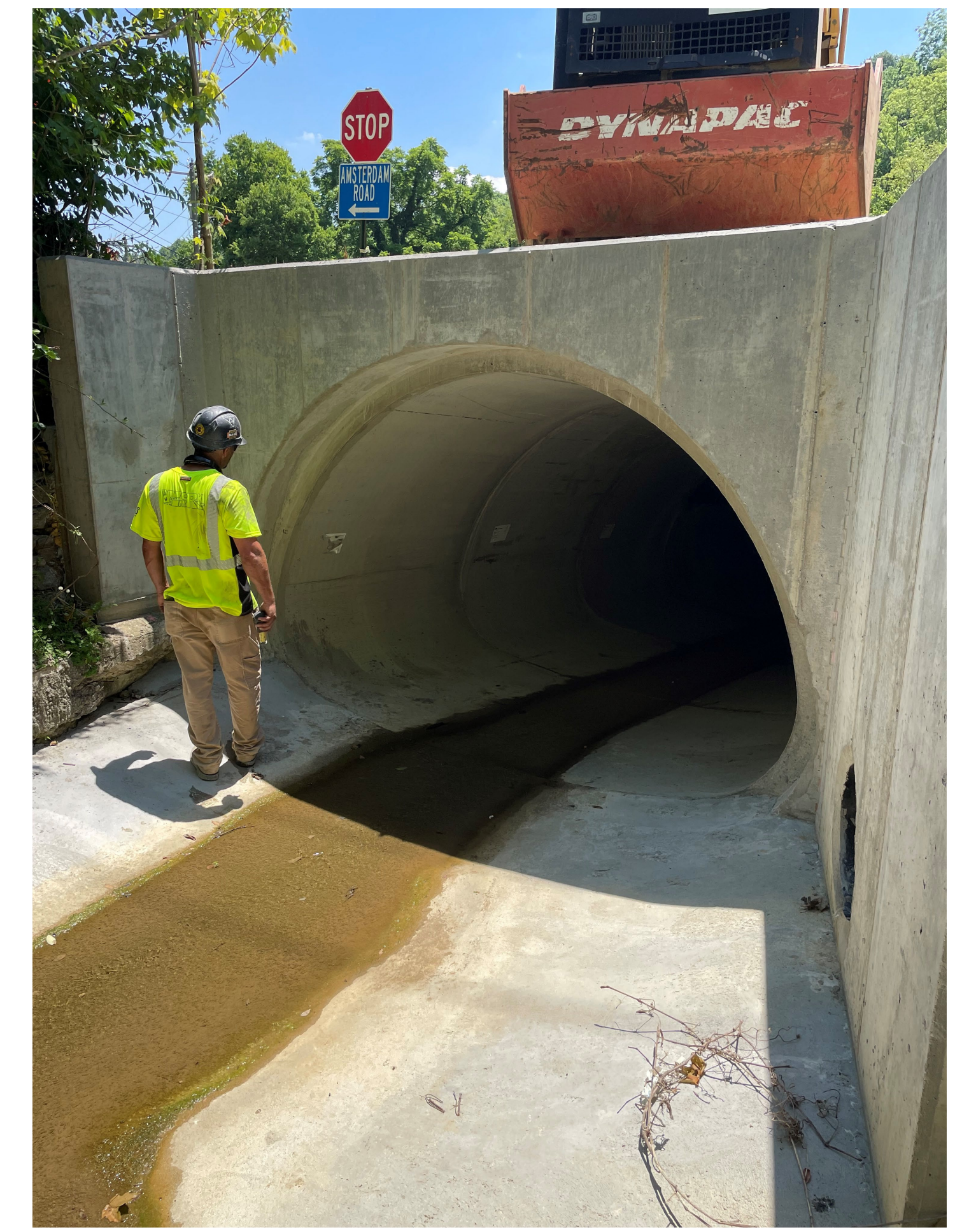
Bromley-Crescent Springs Rd. (KY2373) Kenton Co., KY | 102' of 96" Equivalent Concrete Arch Pipe
