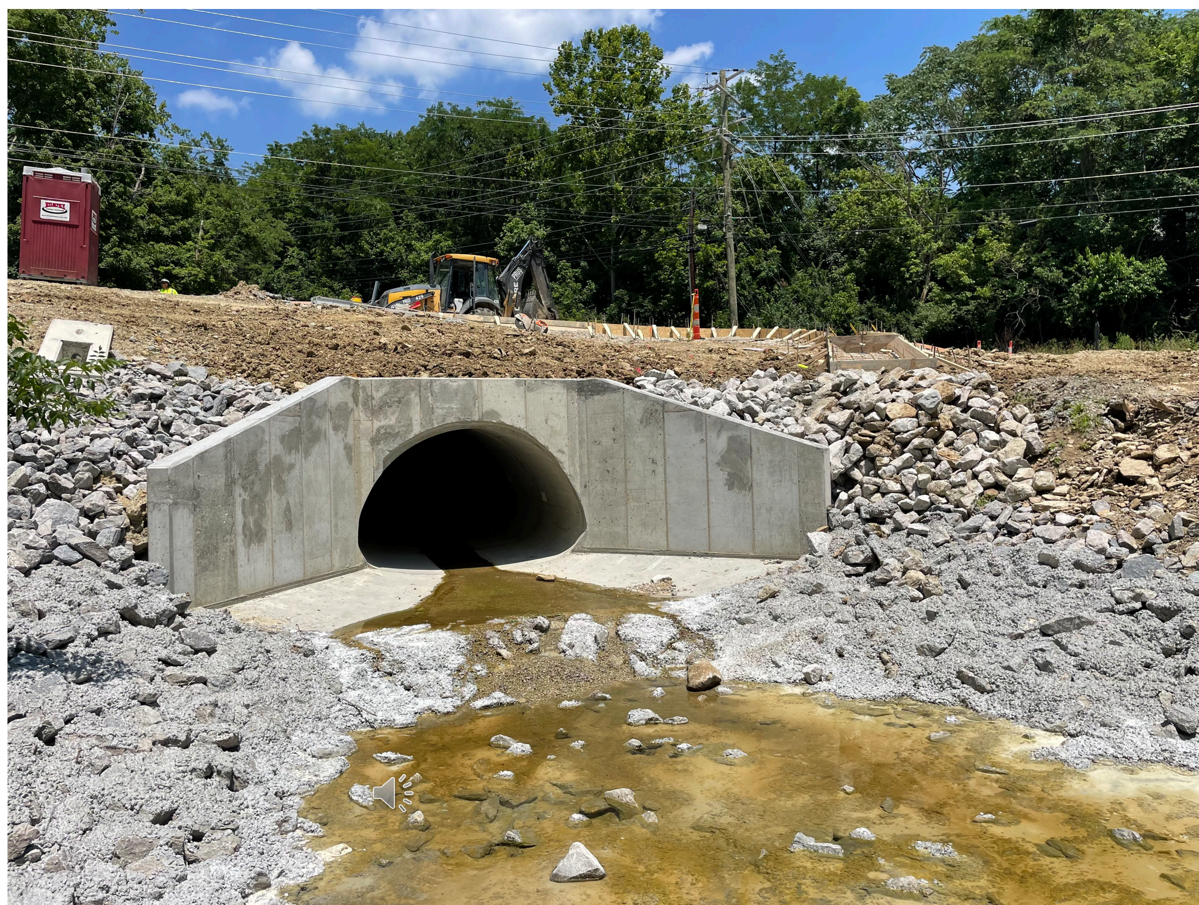
Bromley-Crescent Springs Rd. (KY2373) Kenton Co., KY | 102' of 96" Equivalent Concrete Arch Pipe
