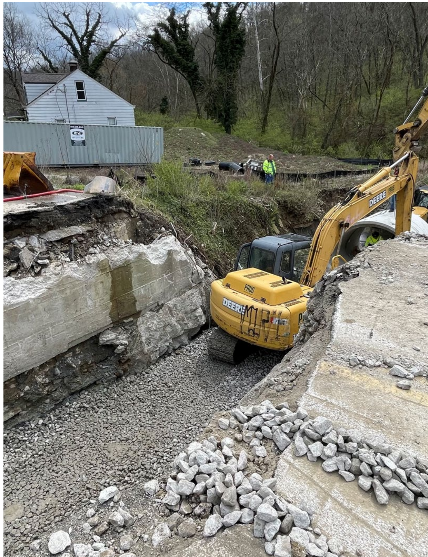
Bromley-Crescent Springs Rd. (KY2373) Kenton Co., KY | 102' of 96" Equivalent Concrete Arch Pipe
