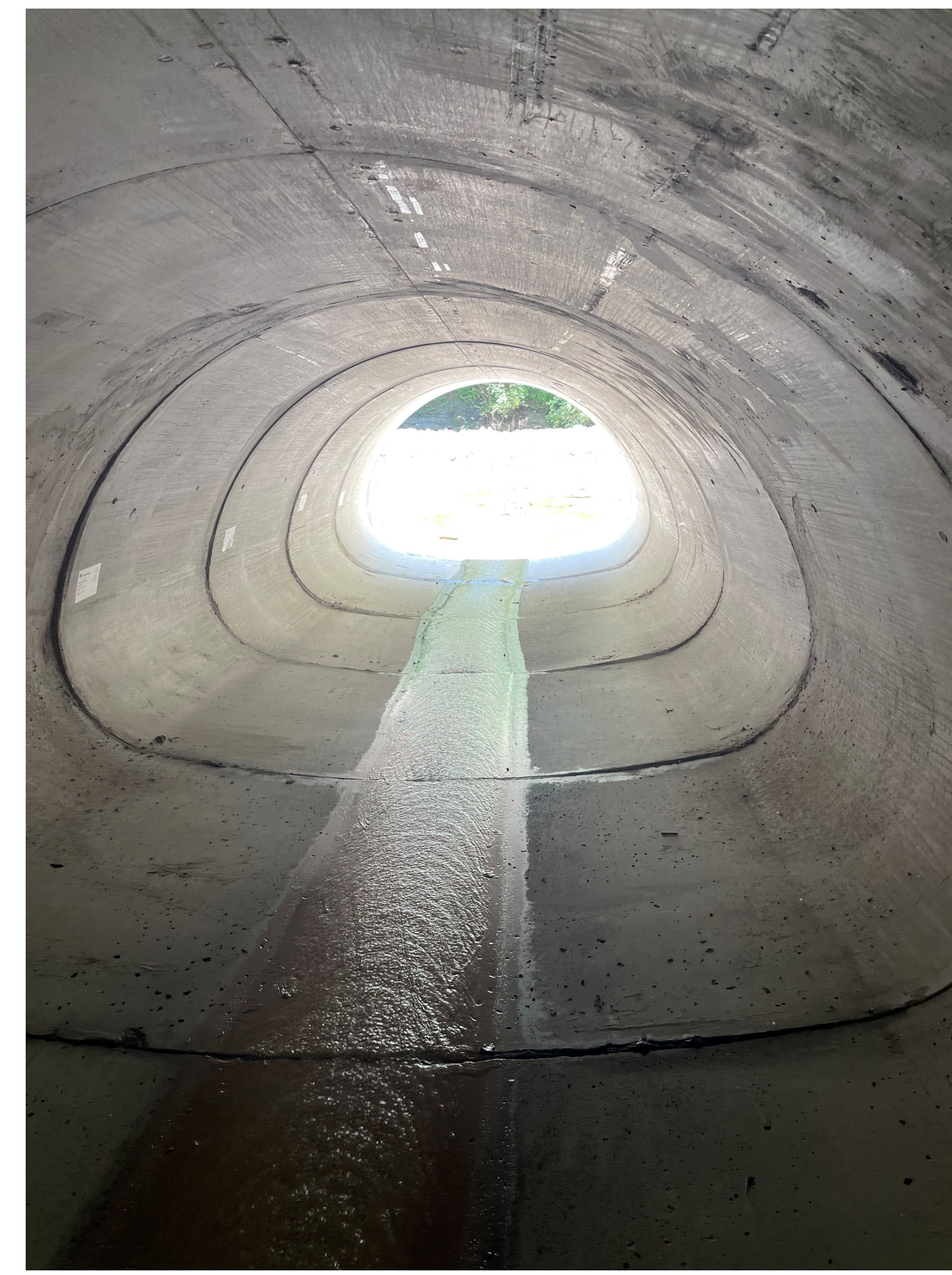
Bromley-Crescent Springs Rd. (KY2373) Kenton Co., KY | 102' of 96" Equivalent Concrete Arch Pipe
