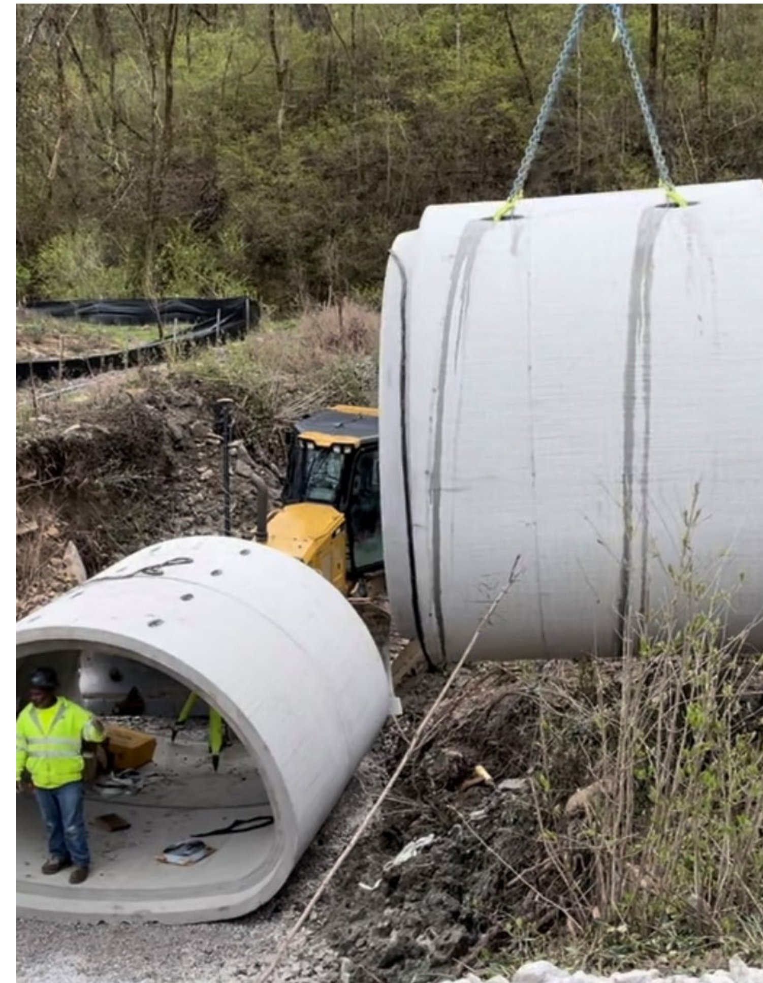
Bromley-Crescent Springs Rd. (KY2373) Kenton Co., KY | 102' of 96" Equivalent Concrete Arch Pipe
